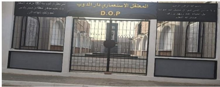
_ Image 02: This photo of Dar Al-Doub detention center was taken after its preparation in June 2024.
